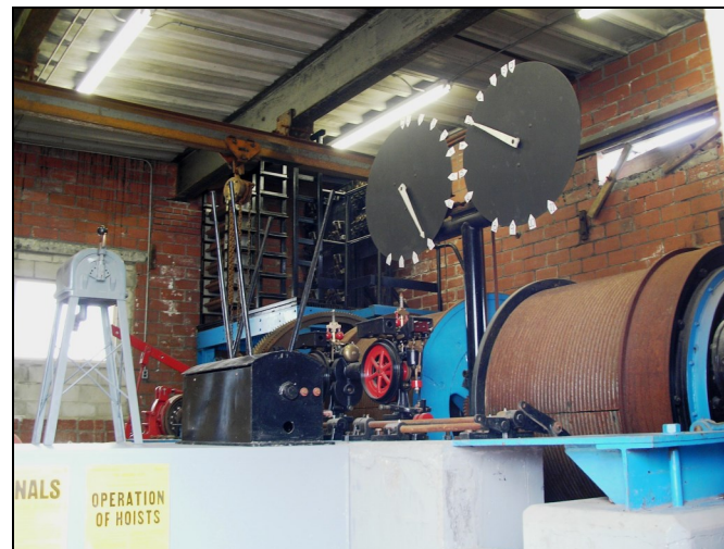
View of Hoistroom Interior
